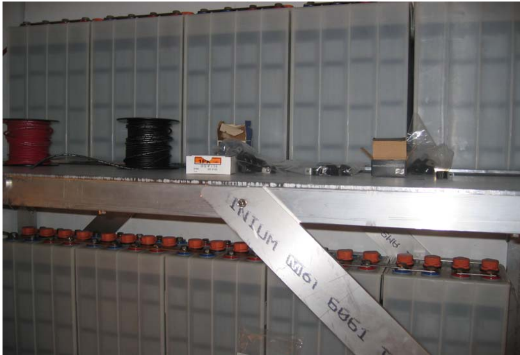
ARRO BATTERY RACK AND SUNICA PLUS NICAD BATTERIES
