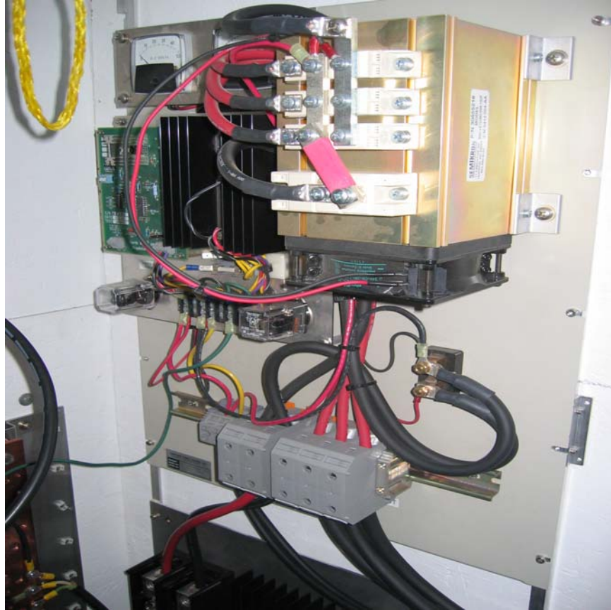
HR3 WIND TURBINE REGULATOR
