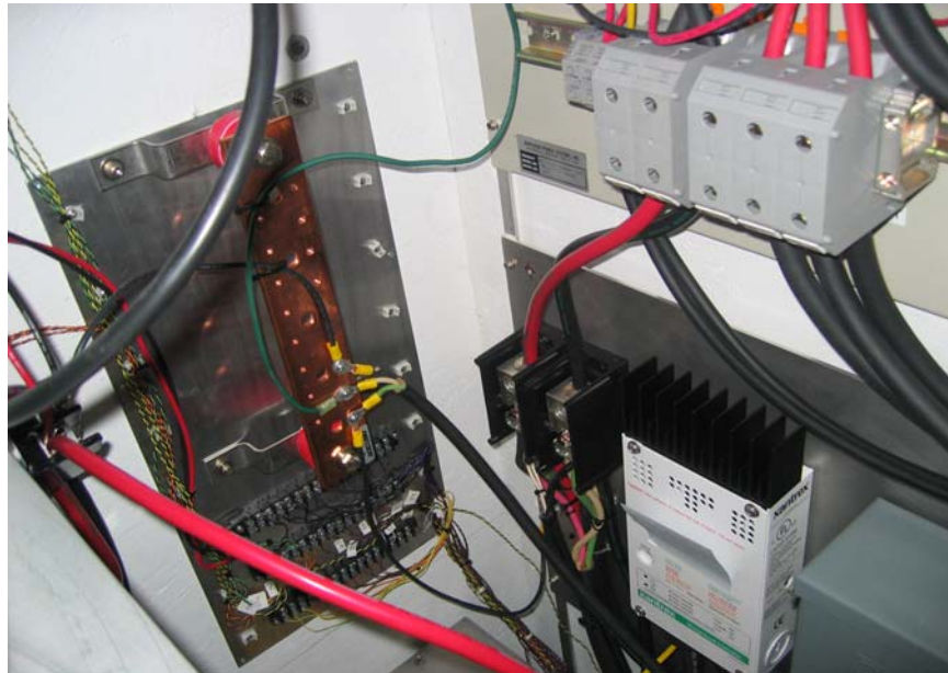
XANTREX COLAR CHARGE CONTROLLER AND TEMPERATURE SENSOR/HEATER BREAKOUT PANEL
